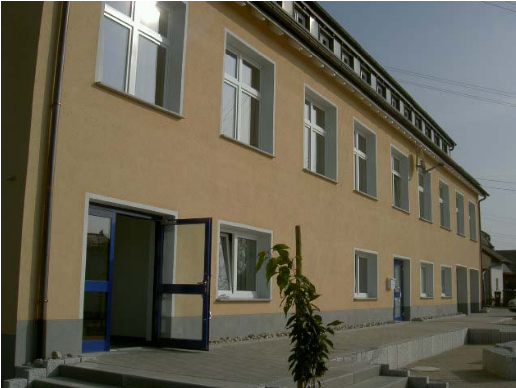
parish hall , Renquishausen
